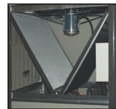
Air-cooled condenser
