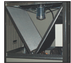
Air-cooled condenser
